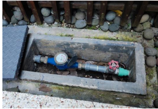
Figure 5. Water Meter Installed in Villa
