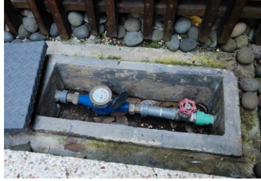
Figure 5. Water Meter Installed in Villa
