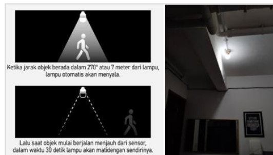
Figure 3. Lights With Motion Sensors in Staff Locker Room
