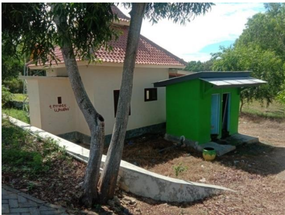
Picture 1: Construction of Mushollaand MCK specifically for cattle travellers. Research Documentation [source]
