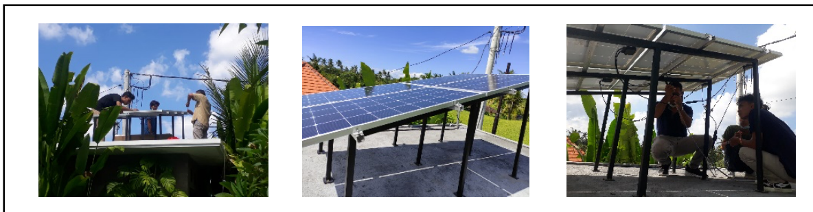
Figure 3 System installation process
