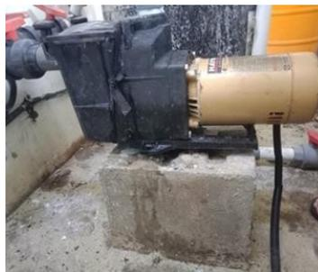
**Figure 11.** Pump foundation
