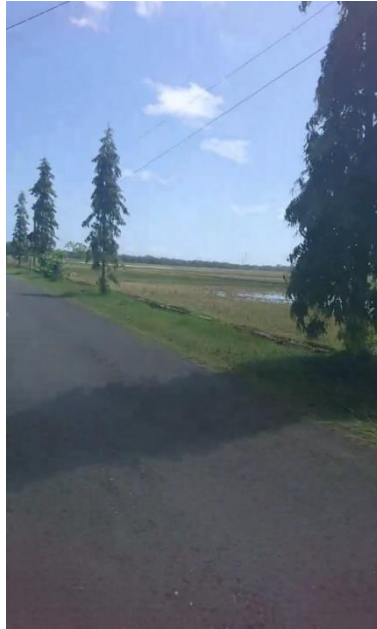
Figure 2. Newest road condition after repaired
