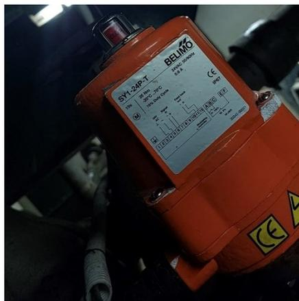
**Gambar 8.** Tampilan kondisi 0% motorized valve
